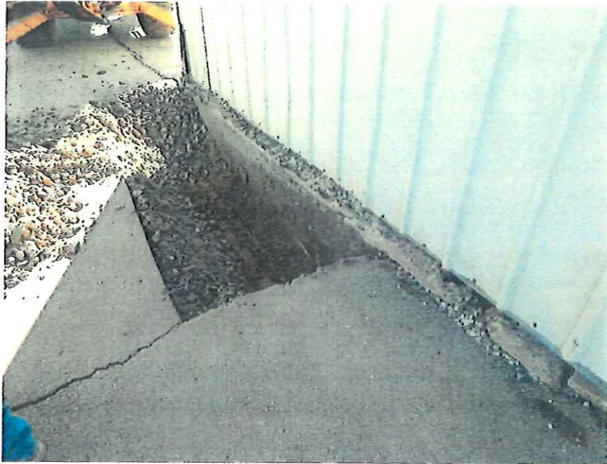
Photo 5. Foundation Wall at Northeast Corner of Building Exposed During Inspection
