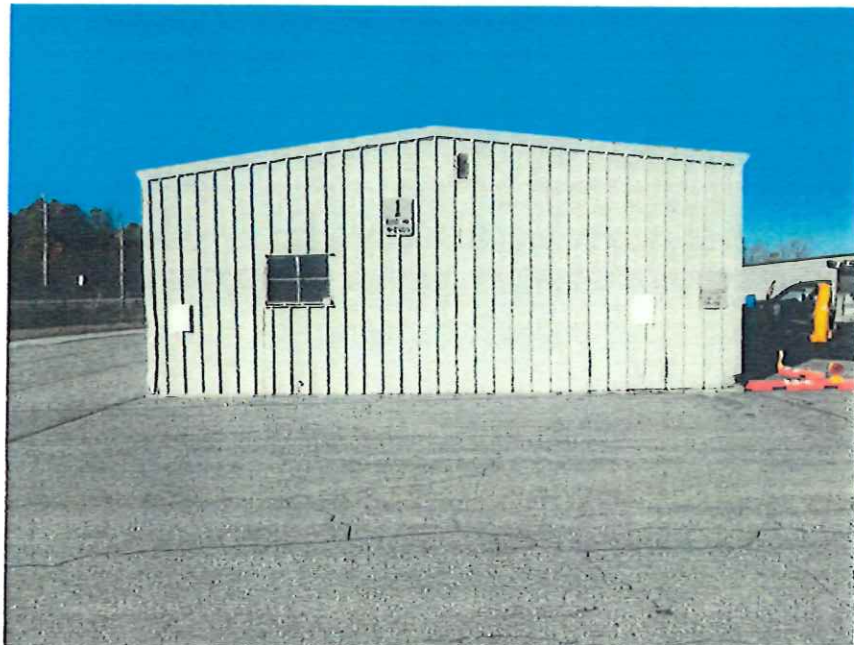
Photo 4. East Elevation of Building
