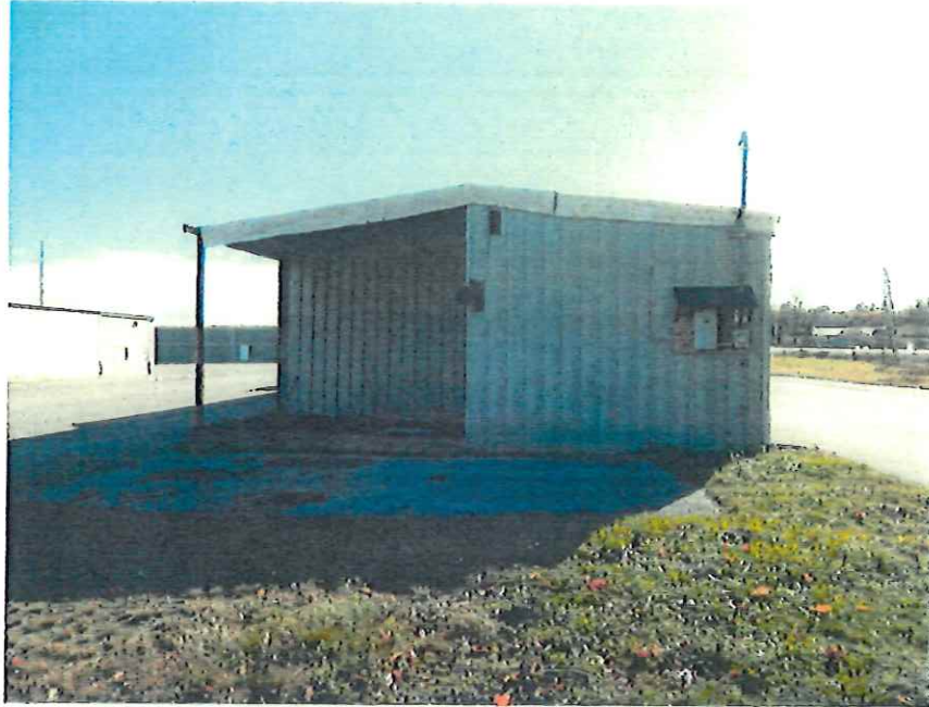
Photo 3. West Elevation of Building
