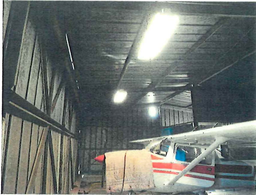
Photo 9. Typical Building Steel Framing at Northeast Corner of Building
