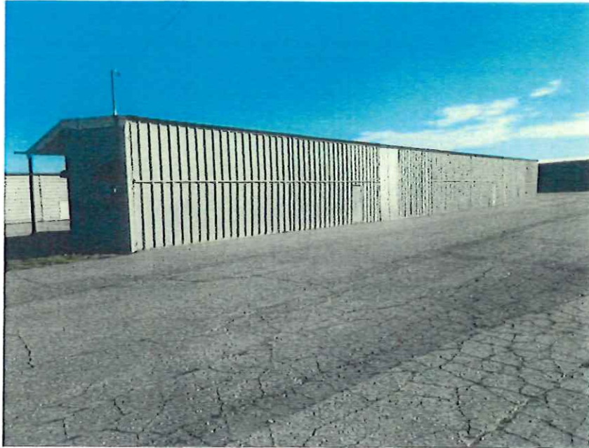
Photo 1. South Elevation of Building
