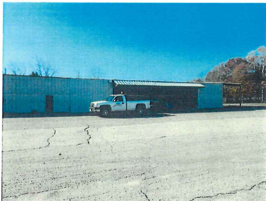
Photo 2. North Elevation of Building
